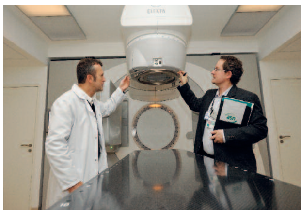
Commissioning inspection of a radiotherapy installation in the Dentellières clinic in Valenciennes – October 2011
